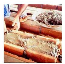
Composite lintels and beams
