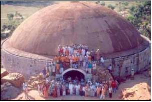
Dome of the Dhyanalingam temple near Coimbatore 22. 16m dia, 7.90m rise, 570 tons – Built in 9 weeks
