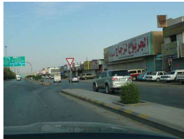
Figure 5.49 Substandard service road access without merging facilities (Prince Saad Bin Abdulrahman Al Awal Rd)
