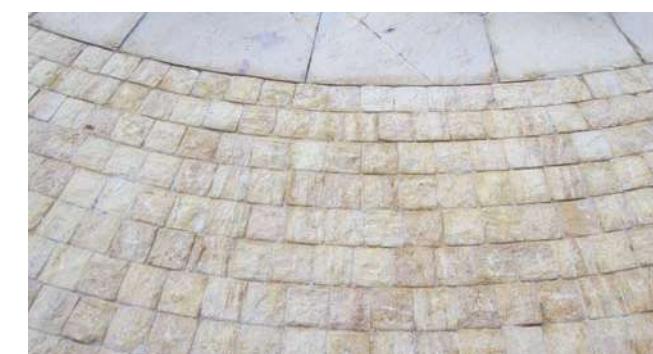
Figure 5.71 Locally sourced Riyadh limestone pavers
