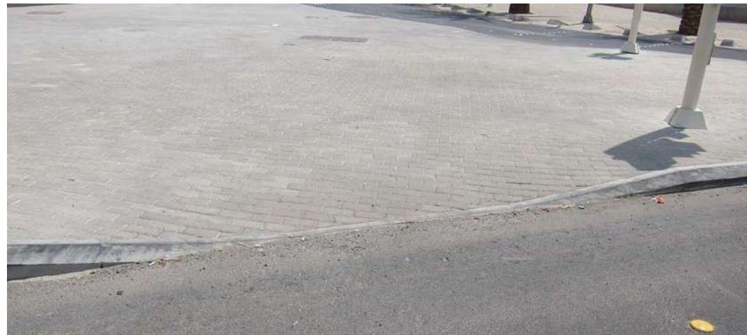
Figure 5.76 Drop-kerb with appropriately sloped walkway, but missing tactile paving – King Abdullah Road
