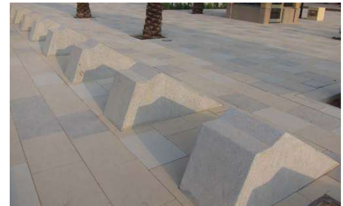
Figure 6.27 Possible security perimeter treatment - Security bollards in front of High Court - Riyadh
