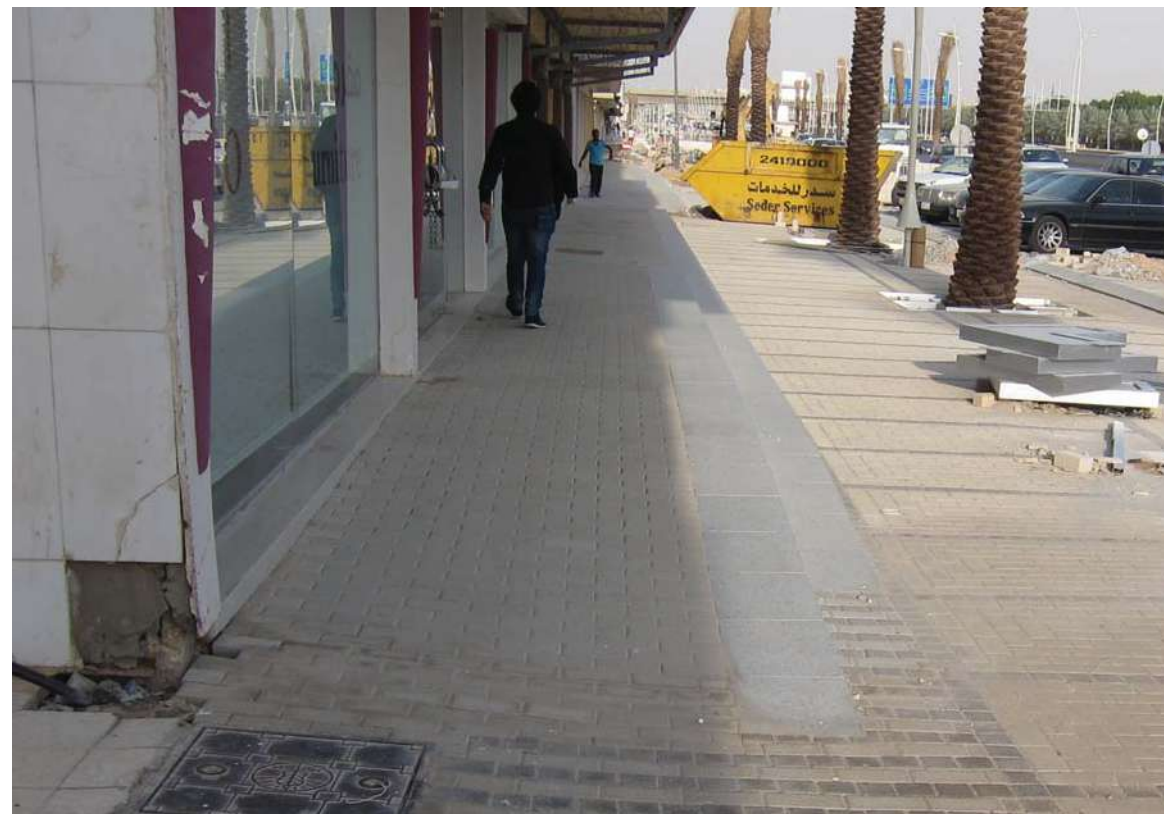
Figure 5.72 Precedent image: Integrated ramped access with steps, allowing wheelchair access to retail units. See detail below.
