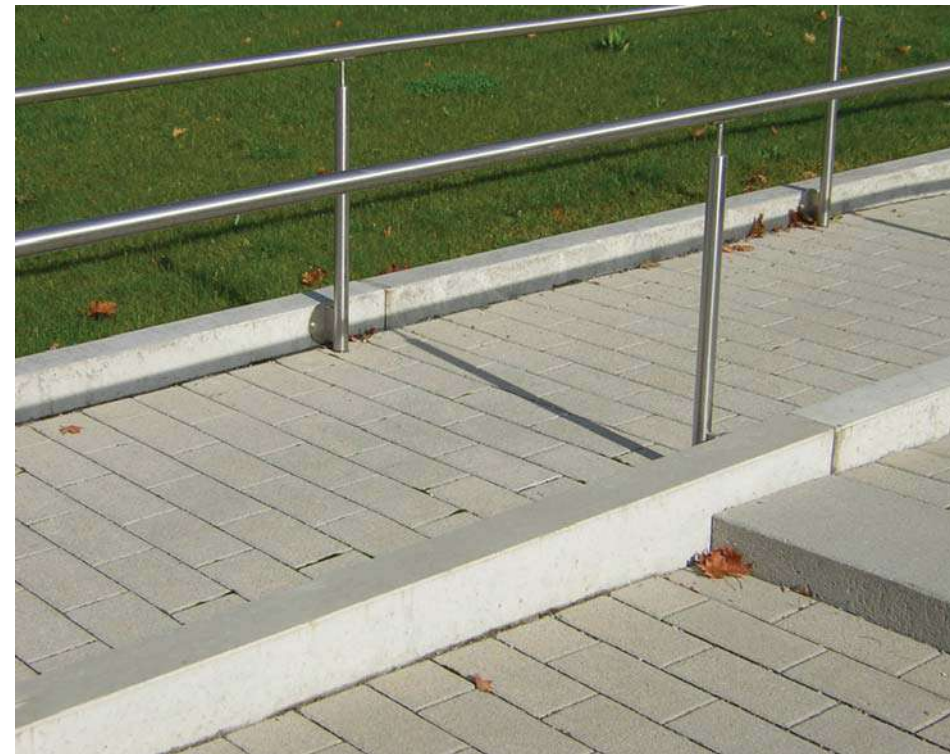
Figure 5.78 Ramp with integrated handrail and upstands to sides
