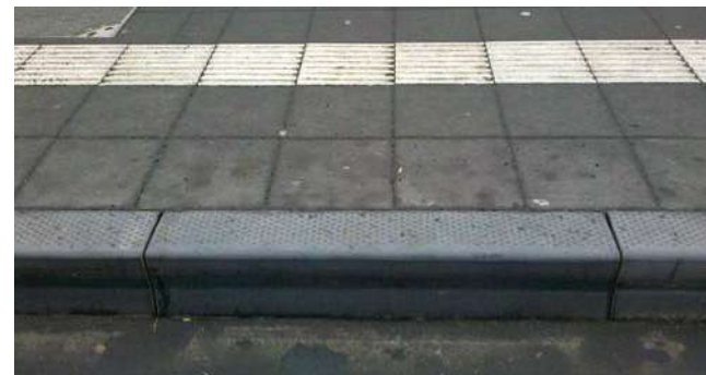
Figure 5.34 Kassel kerb
