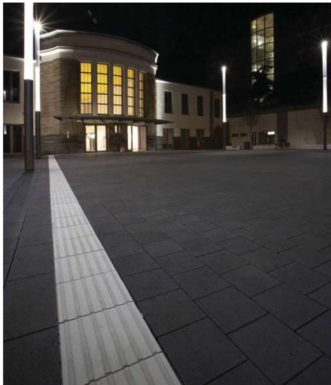
Figure 5.74 Corduroy guidance strip in contrasting tone
