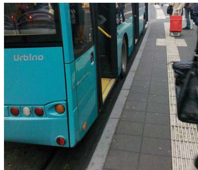
Figure 5.35 Kassel kerb in use at bus stop in Frankfurt
